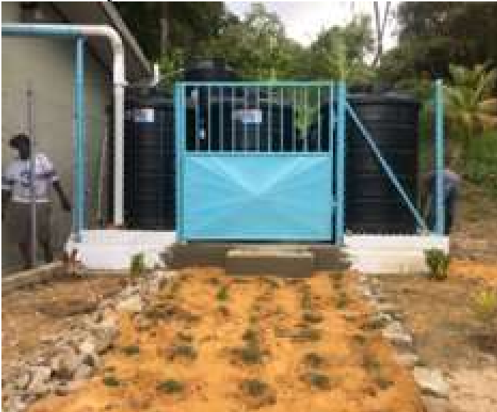
Picture 28: Completed installation of the Rainwater Harvesting Systems at the Cumana Community Centre
